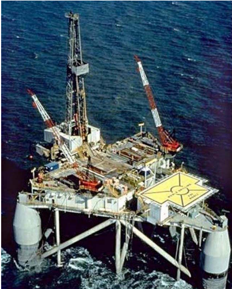
Figure 2: Submersible Drilling Rig (Noble FriRodli) (Reproduced Courtesy of Noble Drilling Corporation)
