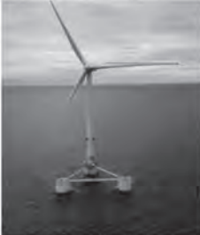
Credit: Photo of the Kincardine Offshore Wind Farm owned courtesy of Principle Power
