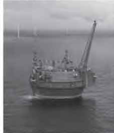
Small Arrays connected to offshore O&G Installations
